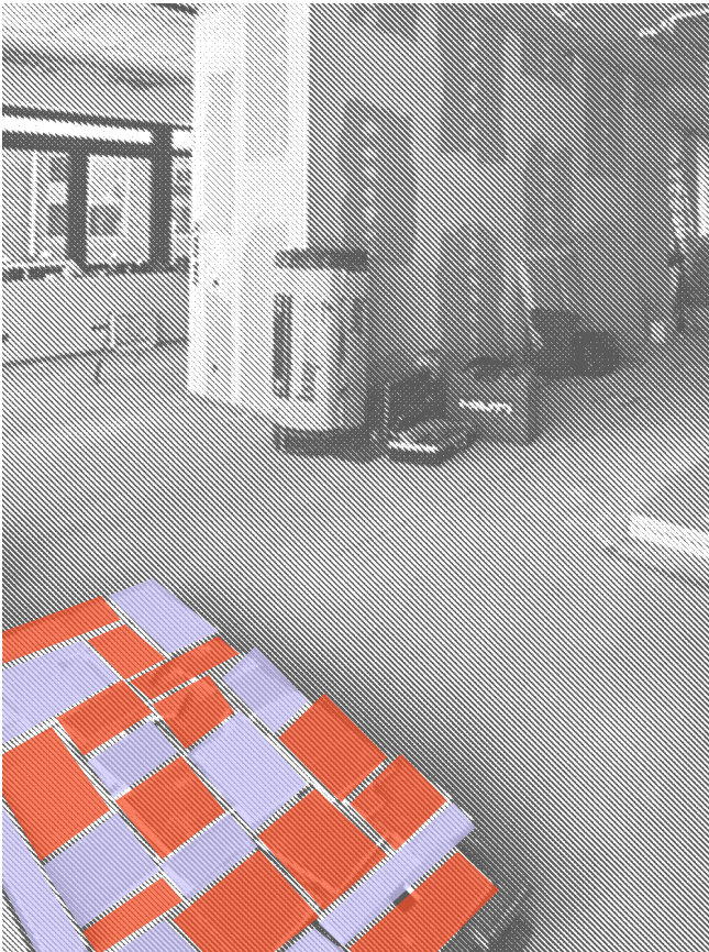
Fig. 07 Small parts were not thrown away, but collected and used wherever possible, for example on the facing bricks of the walls and in the ceiling to create ventilation slots.
